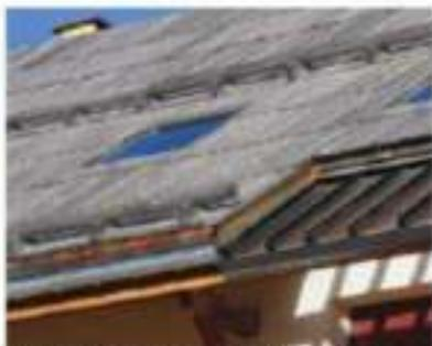
PRINCIPE INSERTION DANS TOITURE BARDEAU
