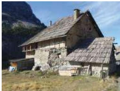
MAÇONNERIE DÉGRADÉE SOUS STRUCTURE À PAN DE BOIS - RISQUE D'AFFAISSEMENT
